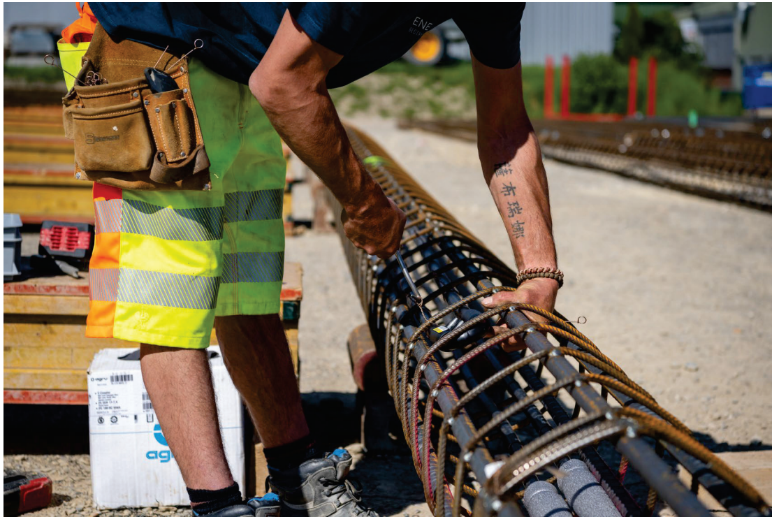
Fixing tubes in the steel cage.
