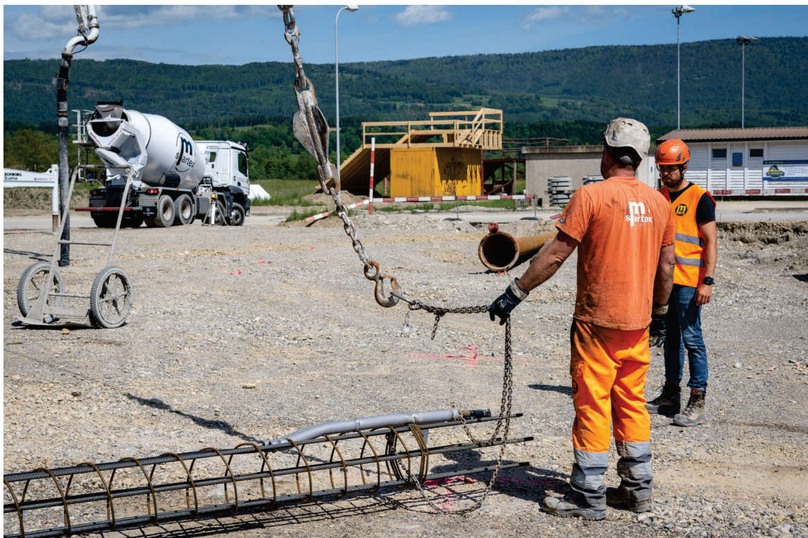
The top of the cage is attached to the crane of the drilling rigs.
