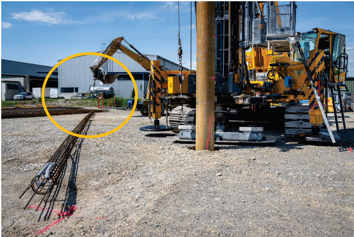
The bottom of the cage is attached to the excavator.
